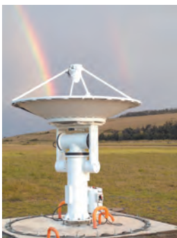
The new Easter Island antenna, under construction.
